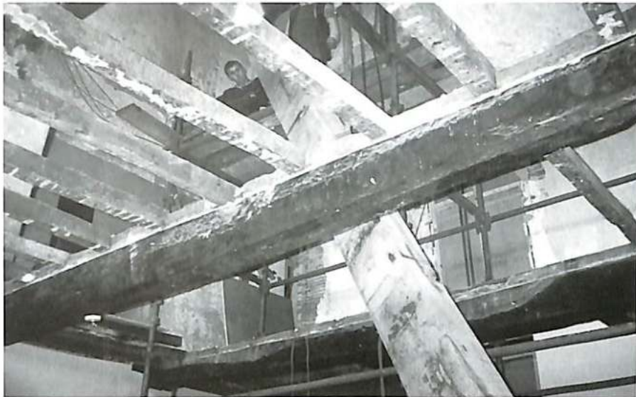
Replacing the oak beam
