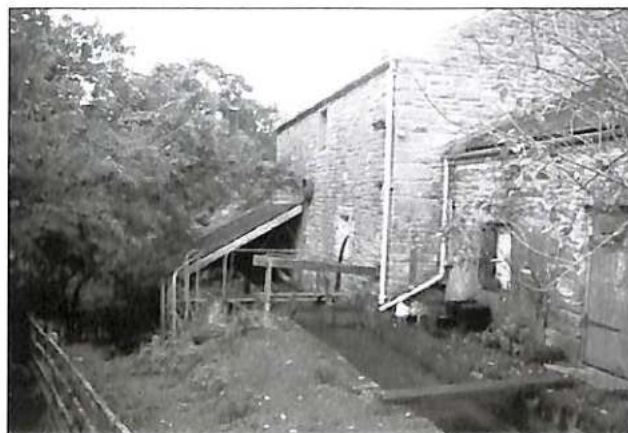
Launder to the twin water wheels at Little Salkeld Mill (DSJ)
