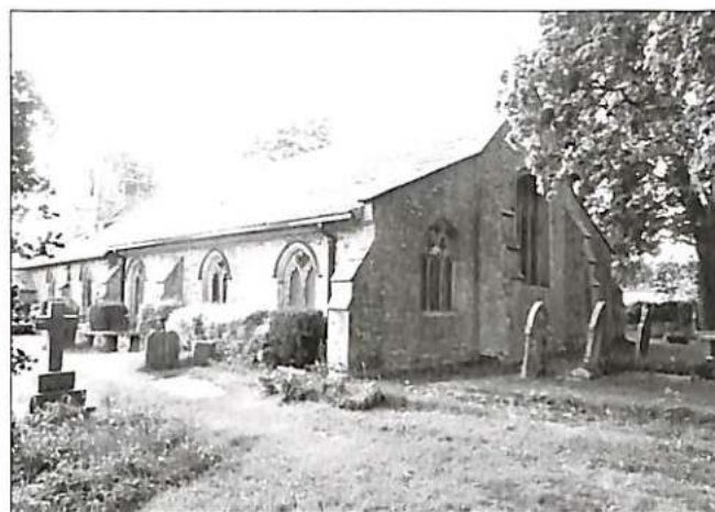
Figure 8 Long Preston church today. Note the more steeply pitched roof and the much more substantial chancel buttresses than before rebuilding
